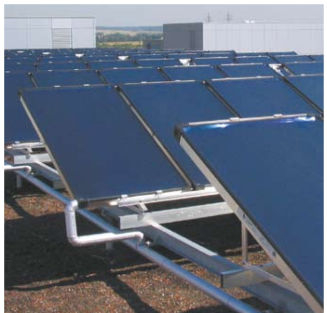
Typical BT collector field
